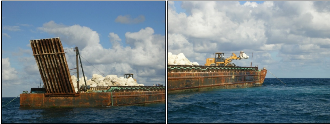
Figure 7. Boulders on the barge prior to deployment at the Golden Beach Reef Site (GDBB) (photos taken 1/10/05).
