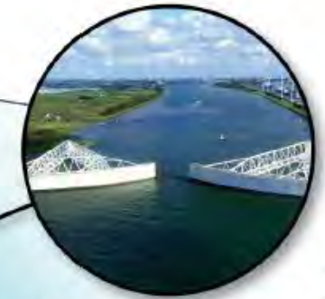
Surge Barrier Gates
